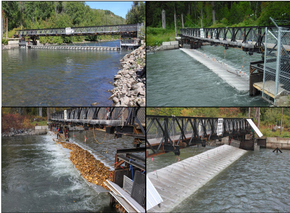
Photo Series 1: The general KSEF structure including fence panels, right and left bank counting stations, overhead walkway, and winch cables suspended from the walkway that raise and lower fence panels according to flow rate and debris build-up.
